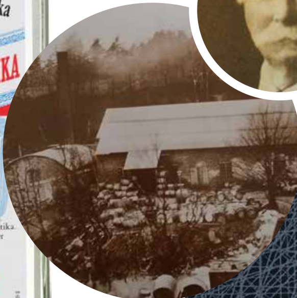
Perstorp's first Formalin plant
