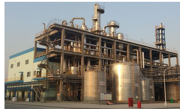
The new Neo plant in operation
