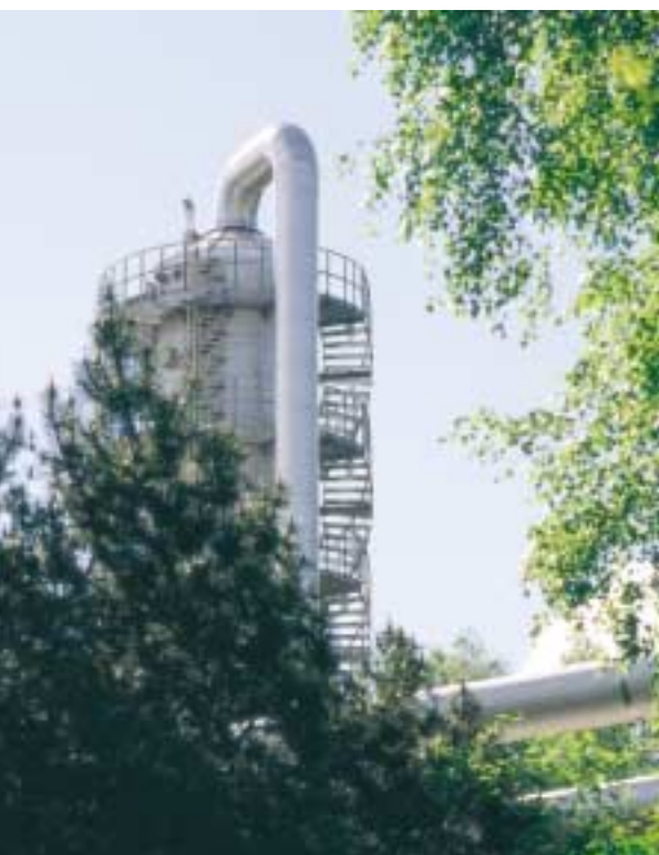
Catalytic incineration equipment is fitted in a large number of plants in order to minimize atmospheric emissions.
