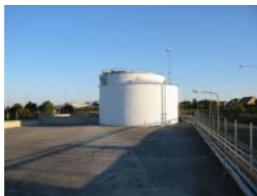
Storage of methanol in the Höganäs harbour.
