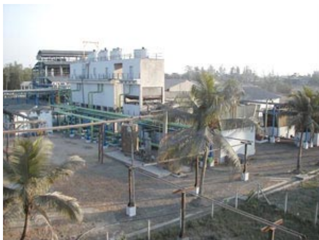
The unit in Vapi, India, with the cooling tower in the middle and the penta factory in the background.
