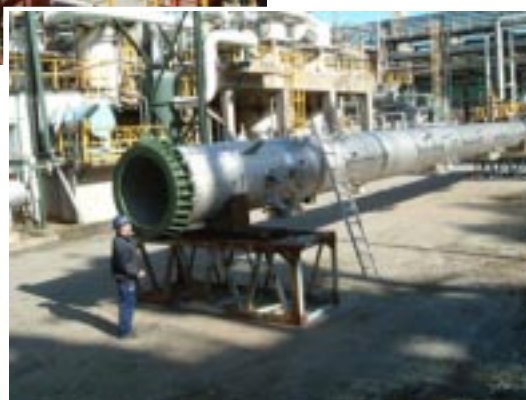
New DEA column in progress at the unit in Stenungsund..
