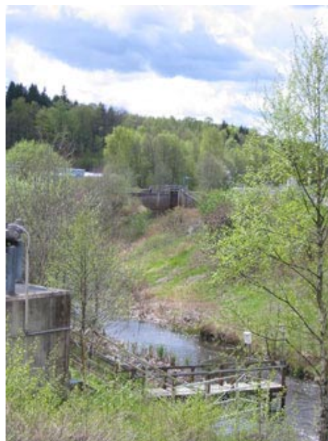
The emergency reservoir has a capacity of 18,200 m 3 .
