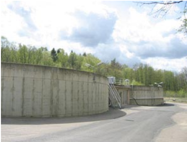
The wastewater treatment plant in Perstorp, Sweden, implemented several improvements and preventive measures during 2002.
