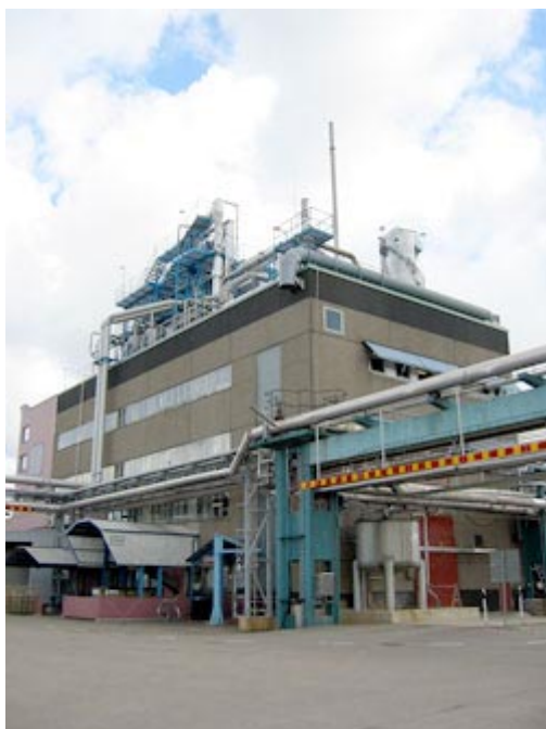
The TMP plant in Perstorp, Sweden, is implementing a project to reduce the consumption of fresh water.
