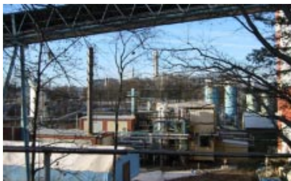
Methanol from the polyol production plant at the unit in Perstorp, Sweden, is conveyed to the formic acid plant for thermal incineration, replacing oil.
