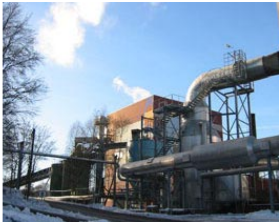
Bottom ash and flyash occur at the steam power plant in Perstorp, Sweden, operated by Perstorp Support AB. Most of the flyash is reused within the concrete industry.
