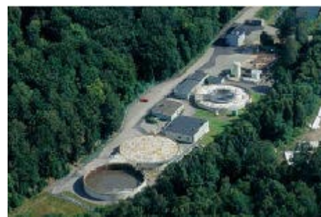
Wastewater treatment plant in Perstorp, Sweden
