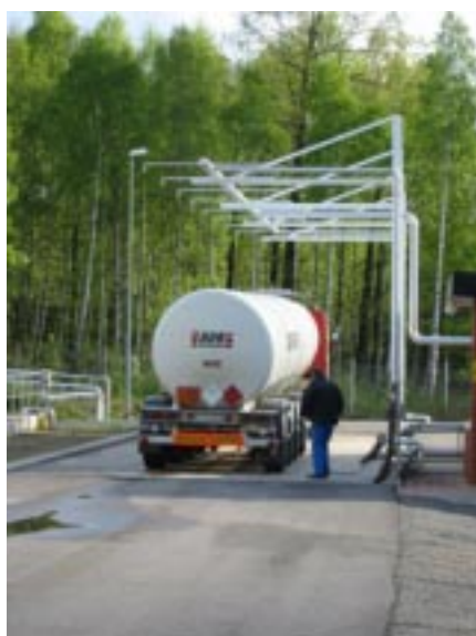
Unloading of methanol at the site in Perstorp, Sweden.
