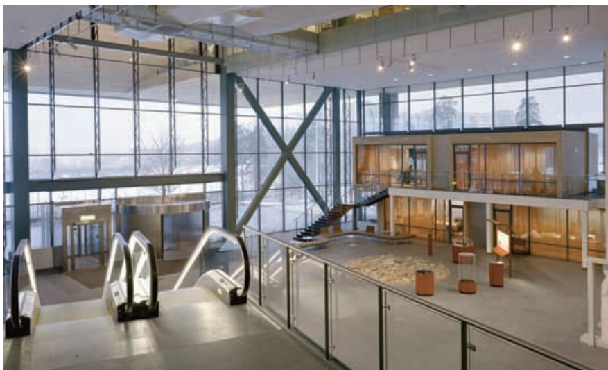
Steel components covered with paint containing Charmor in the binding agent mean that, in the event of fire, people have more time to evacuate a building. See the section Product Stewardship on page 12.
