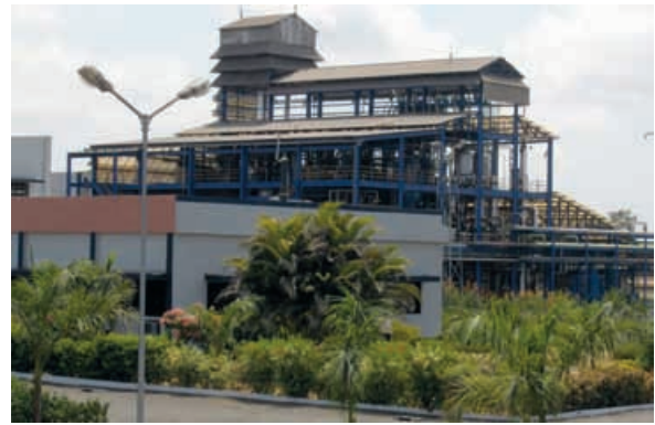
One of the three boilers at Perstorp Aegis Chemicals in Vapi, India, was converted to use a bio-fuel system with excellent results. Emissions of sulfur dioxide have been drastically cut because the plant now burns briquettes made from bagasse, which is a waste product from the sugar-cane industry.
