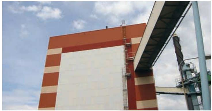
The steam power plant at the largest company site in Perstorp, Sweden, supplies steam and electricity to the entire Perstorp Industrial Park. The switch from coal to biofuel took place in 1991. The main fuels are wood chips, demolition wood and peat.
